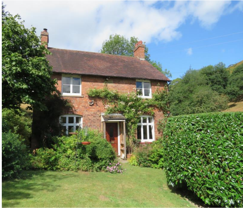
Reservoir Cottage, Batch Valley
